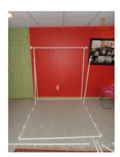
Insert the two 45" tubes in to the first two two tees and attach two tees on the top.
