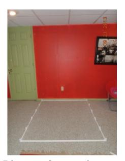
Step First is to build the base. For the four corners you need the side elbows; On the front and back use two 51" pipes; on each side use five 10" pipes; between the 10 " pipes, install tees (8 in total). Snugly fit the pipes together, with the open outlet of the tee upwards. Use the hammer to lightly tap the pipes and fitting together, but do not force them all the way in. You will need some space to adjust for any variations in cutting.
