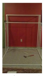
Complete the second step with one 51" pipe and two 10" pipe. Level in both directions and tap in the pipes if necessary
