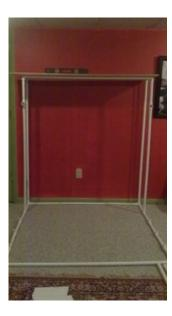
Ensure the first step is in level on both directions. Tap the pipes slightly to get them in level – go gently as you will need the play room for final fitting.
