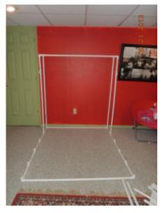
Insert 9" pipe on top each of the tees on the 45" pipe. Insert side elbows on top of each of thees 9" pipes; complete the first step frame with two 9" pipe and one 51″ pipe.
